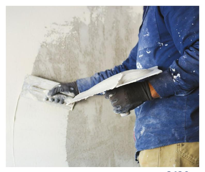
**G120**Cementitious Adhesive for Thermal Insulation Boards
